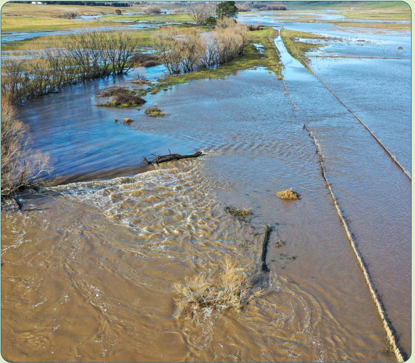
Mulloon Home Farm flooding, 2022
